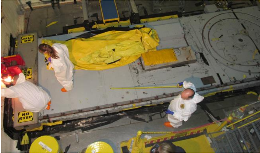
Figure 2.13: Workers Operating the Portable Maintenance Shield [35].
