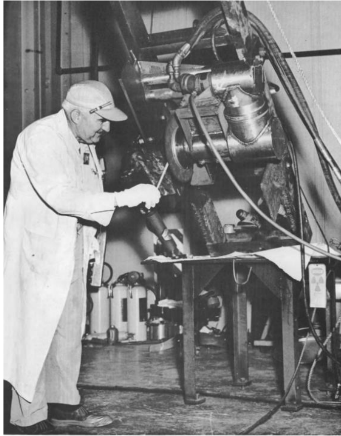
Figure 2.5: Dismantling of the ARE Reactor Core through Cutting [30].
