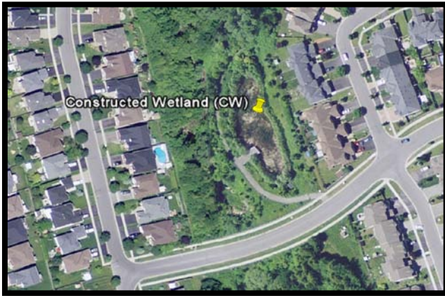
Figure B1. Constructed Wetland (CW) in Early Spring
