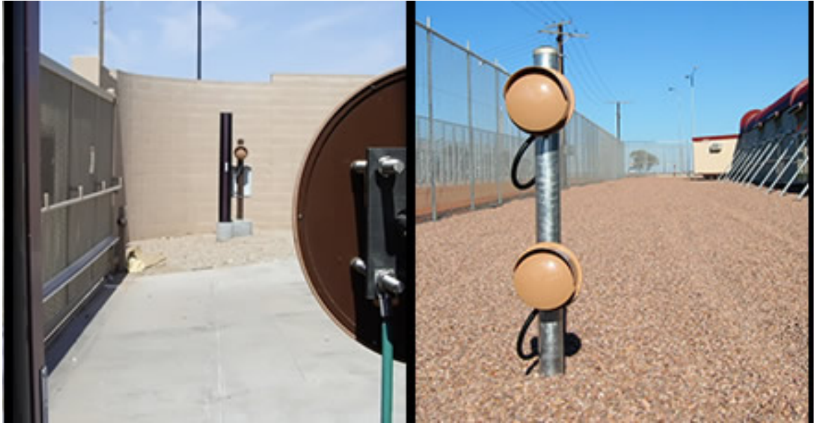
Figure 3.2: microwave detectors, left is bistatic, right a monostatic [31].
