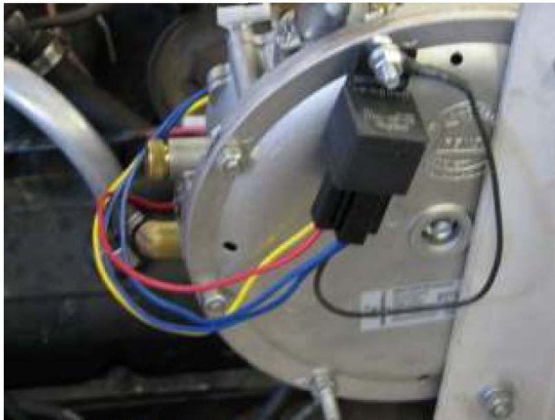
Figure 3.5: Relay with all wires connected behind the regulator.
